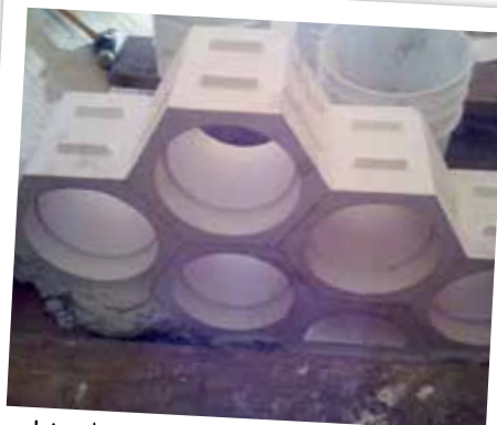
blocks are locked together at installation
