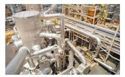
and footprint. New installations may also benefit from using standard design vessel sizes with element blank offs for future expansion capability.
